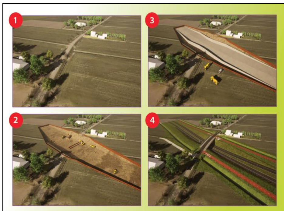
Figure 29. Overview of the Middelberterweg underpass.
