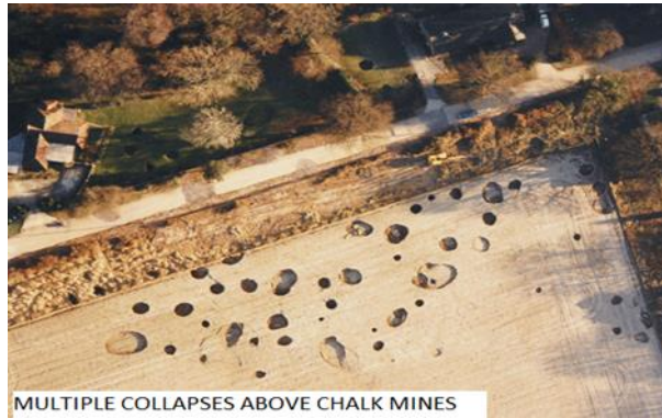
d) Surface collapse above chalk mines.
