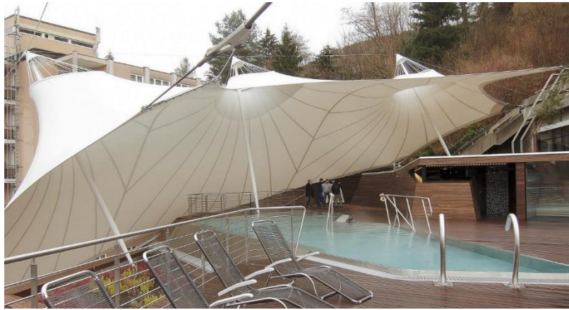
Figure 3.7 The membrane structure Palais Thermal Bad Wildbad.
