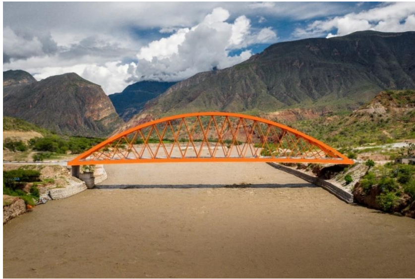
Figure 3.6 Bow-string bridge with inclined, prestressed hangers.
